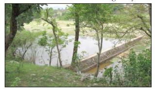
dams, contour trenches, and field bandings all prevent the monsoon rains from flowing down the hills at a destructive velocity. These three structures, constructed on different areas of land, increase soil moisture, increase se water tables in the area, help recharge nearby and downstream wells, and directly contribute to agricultural productivity by
